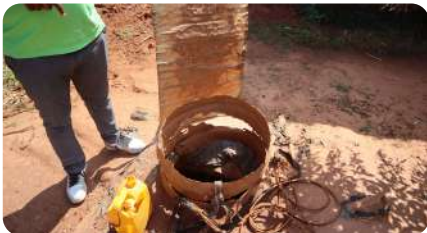
Local operator exposing technical details of damaged borehole to be restore thanks to the project
