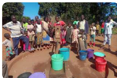
People filling water cans using rehabilitated boreholes
